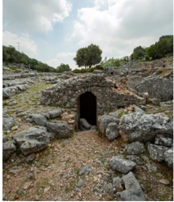
A cistern on the Via Sebaste
